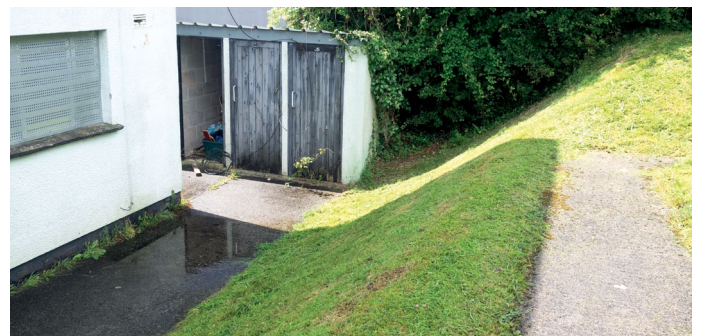
Images 4 & 5: Lack of surface water management means the risk of flooding is high on such a steep development
